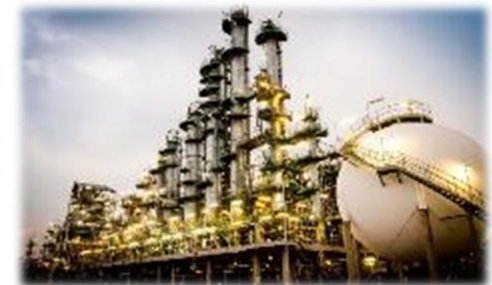
Baker Hughes turbomachinery is installed at many industrial complexes around the world
