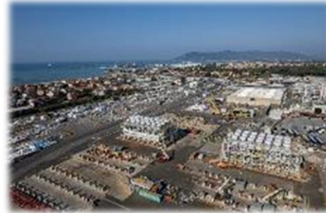
Modules under construction at Baker Hughes' Avenza facility in Italy
