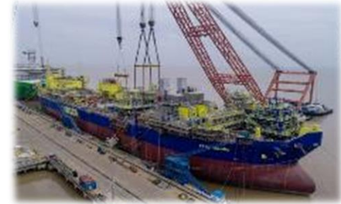
Baker Hughes equipment being installed on an FPSO
